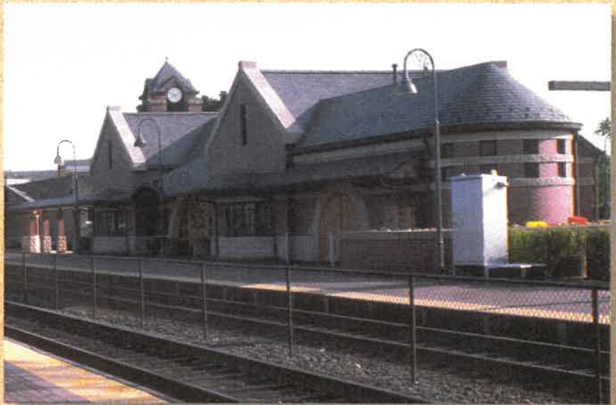
The Metra train station in downtown Glenview, an award-winning design
