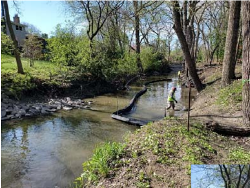
Slope stabilization and rock toe
