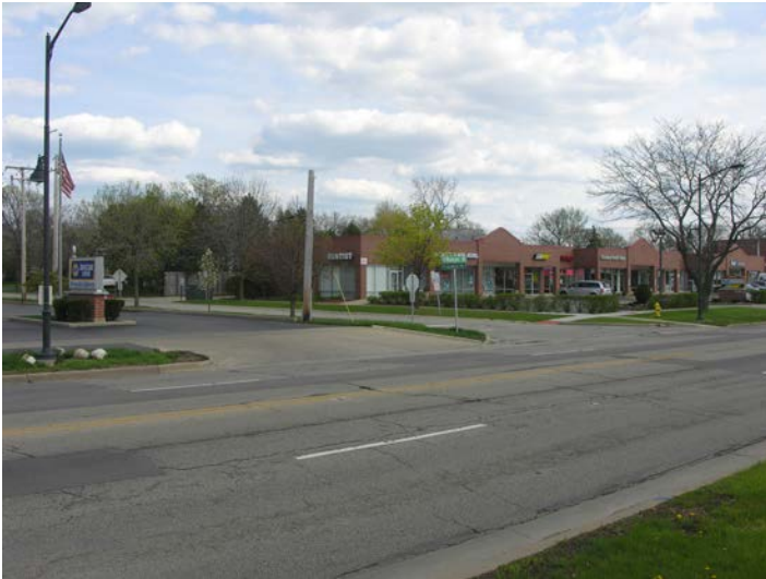
Access too close to intersection. NAPA Auto Center entrance too close to Glenwood Ave.
