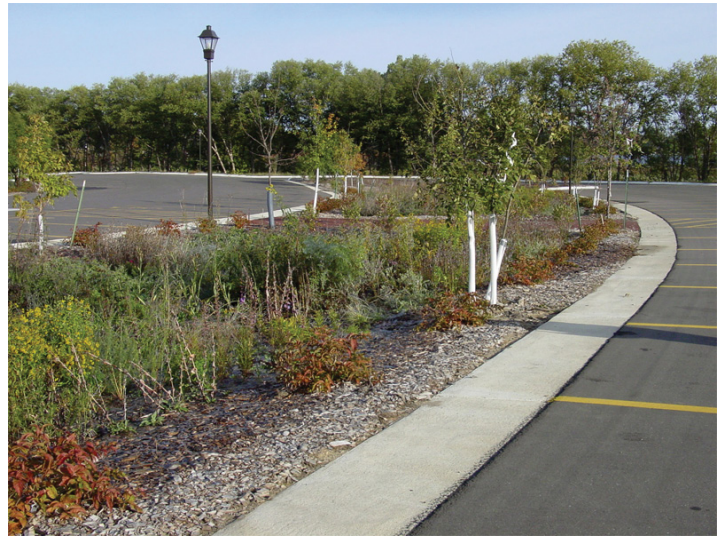
Various green technologies can be employed to increase natural water retention and reduce runoff.
