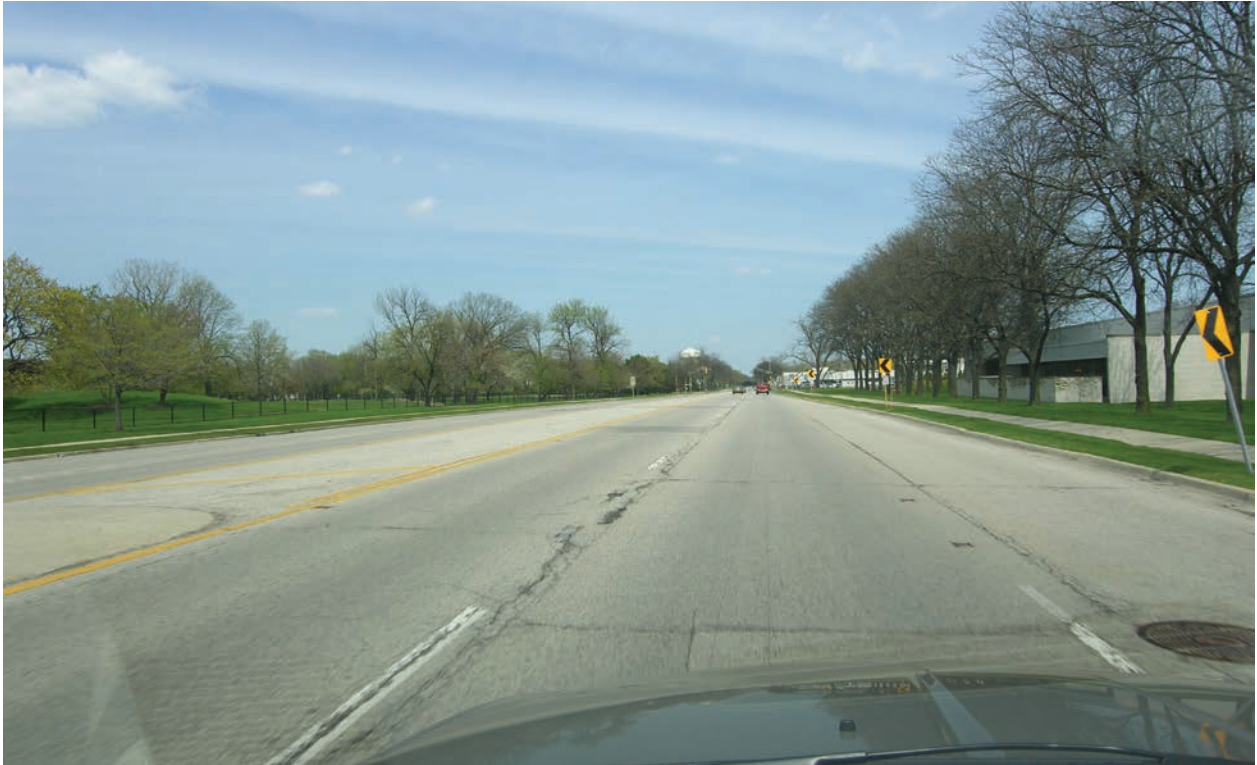
Existing Conditions. Looking north along Waukegan, north of Golf.
