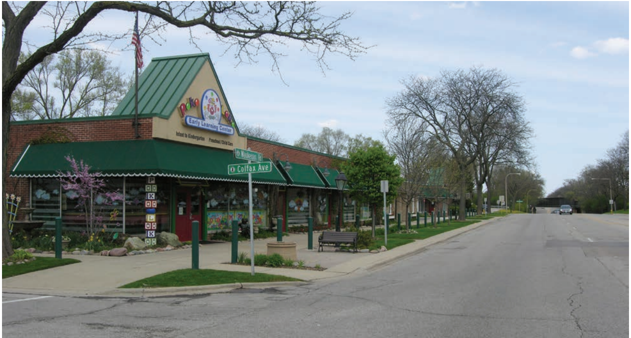
Existing Conditions: Looking north along Waukegan from Colfax towards Harrison. No separation between Waukegan and day-care pick-up and drop-off.
