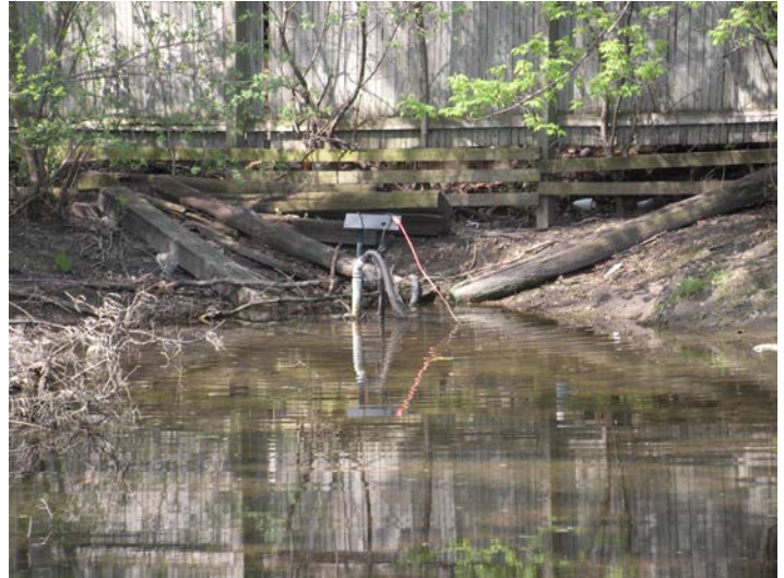
Pumping of standing water. Behind Loren Hyundai.
