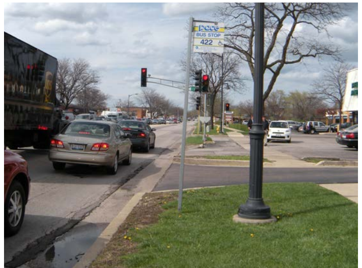
Inadequate bus stop facility. Taco Bell looking north along Waukegan towards Chestnut.
