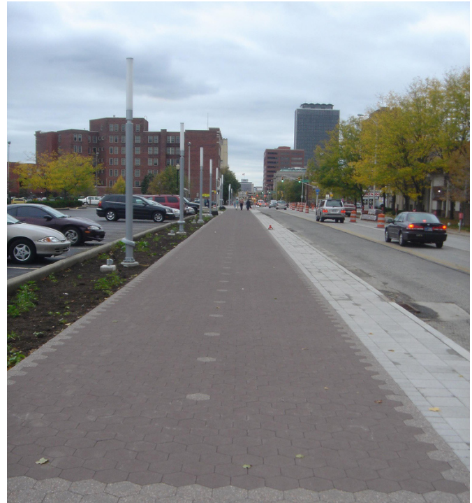
Sidewalks should be widened into a 8-10 foot multi-purpose path to accommodate both pedestrians and bicycle.
