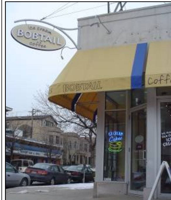
Blade sign is attached with wiring from the roof (4a1)
