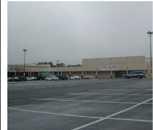
A large parking area that has no landscaping islands or trees (1) (Courtesy of the Coalition for Smart Growth)
