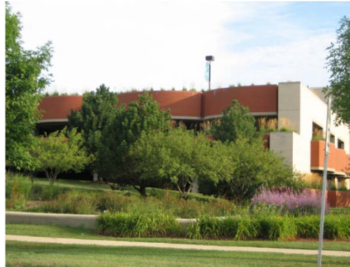
Parking lot perimeter is landscaped at ground level (3)
