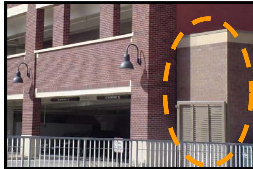
(2). Equipment is shielded from the right-of-way with a masonry structure attached to a parking garage.
