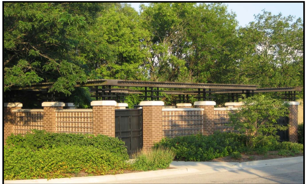
Dumpsters and utilities are suitably screened in a parking lot with an architectural wall, solid metal gate and a mixture of landscaping materials.
