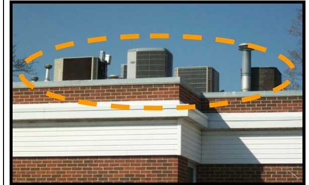
(1). These mechanical units could be blocked from public view with compatible architectural screening.
