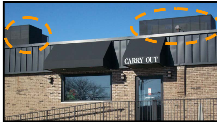
(1). Mechanical units are screened from the view of the parking lot using awning fabric to blend with the mansard roof.
