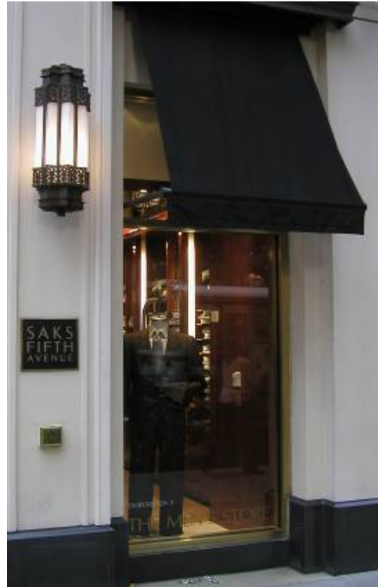
Well-maintained awnings, constructed of architectural fabric, in a matte finish (3.1 & 3.4)
