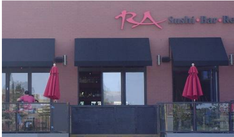
Projection over individual openings of the façade (1.1)
