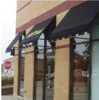
Multiple awnings reflect window openings (1a)
