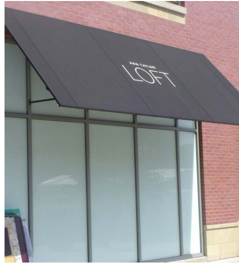
Text and graphics shall comprise no more than 20% of the total awning surface (2.1)
