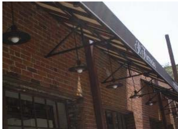
Decorative under-canopy lighting may be permitted but requires Appearance Commission review (4c)
