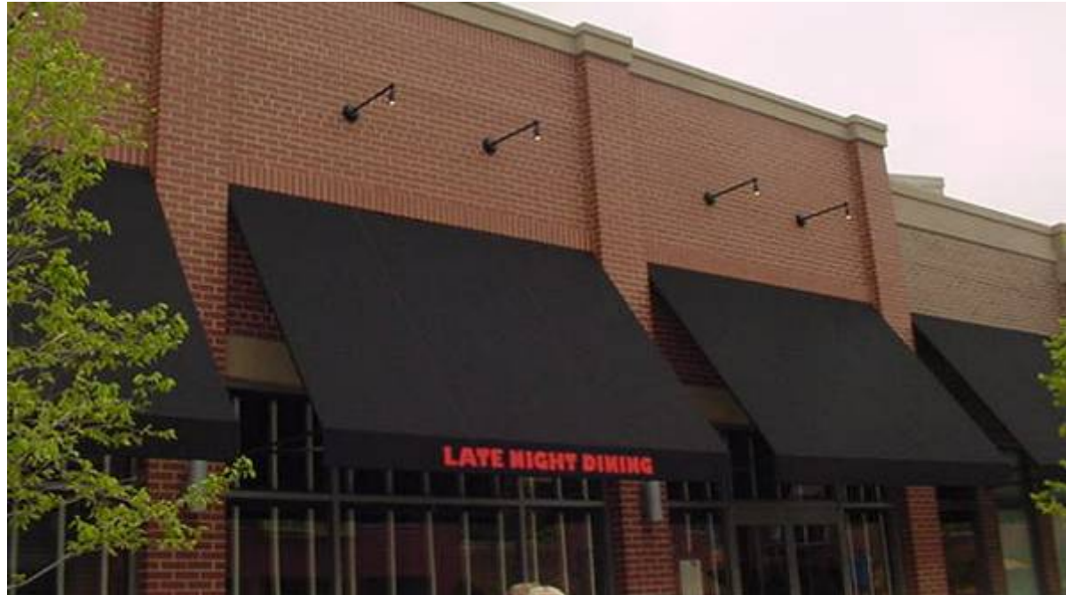
Appropriately spaced lighting fixtures provide a wash of illumination on the awning (4b)
