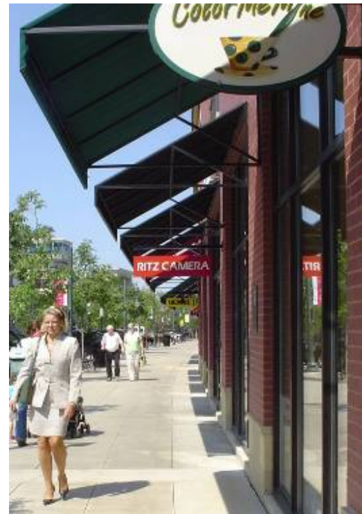
Lowest point of the awning is a minimum of 8' above the ground (1.2)
