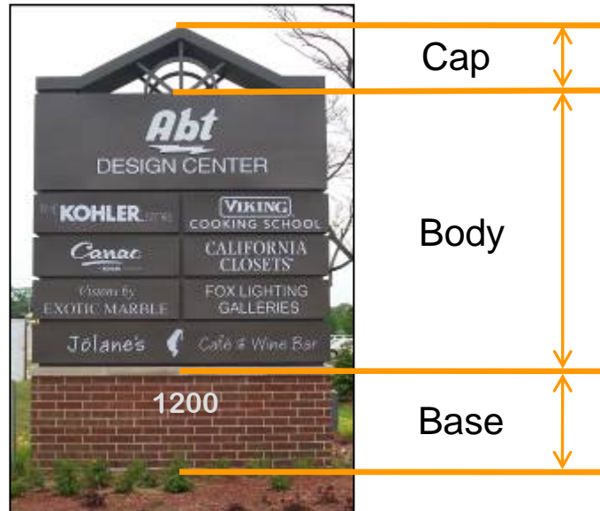
iva - Sign base provides at least 1' height
