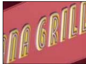
iv2 - Push-thru or routed out letters & graphics are encouraged to provide dimension
