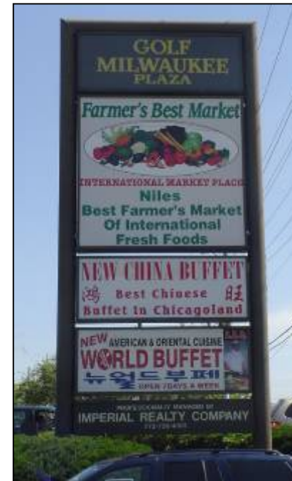
iva - Sign does not have an adequate base
