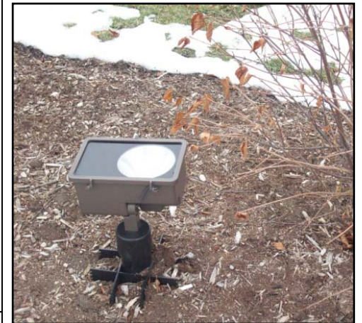
(a)(1) Lighting could be shielded or changed to a directional spotlight to avoid light spill into the night sky.
