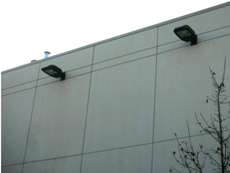
Security lighting for nighttime safety that directs light down rather than out.
