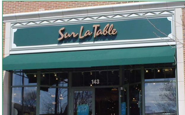
Contrasting, non-illuminated pin letters maintain the character of the existing storefront façade (2c)
