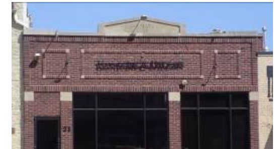
Pin-mounted letterforms should contrast with the background material, not blend in so that the sign is illegible (2c)
