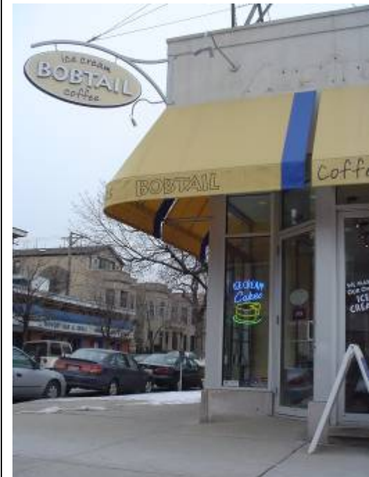
Blade sign is attached with wiring from the roof and is oriented toward automobile traffic (4a1)
